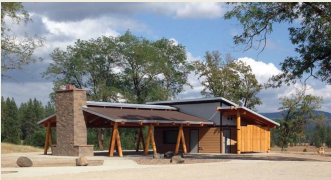
Spokane Indian Housing Authority Community Pavillion, Photo: Kari Hutchison
