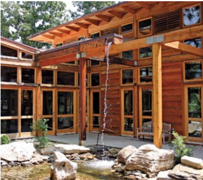
The Bernheim Arboretum Research and Visitors' Center used reclaimed materials, mechanical connections and reconfigurable modules to reduce waste and greenhouse gas emissions. Photo: Lifecycle Building Challenge via William McDonough + Partners
