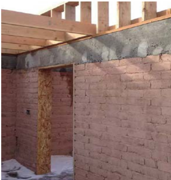
The Apsaalooke Crow Tribe used Crow resources and tribal member labor to build compressed earth block homes. Photo: Apsaalooke Housing Authority
