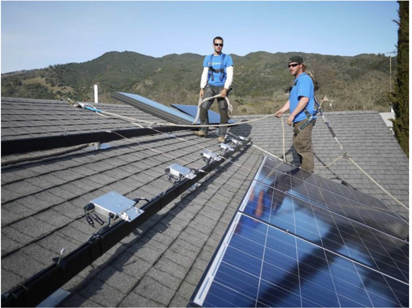
Grid Alternatives Solar Installation, Hopland Band of Pomo Indians, California
