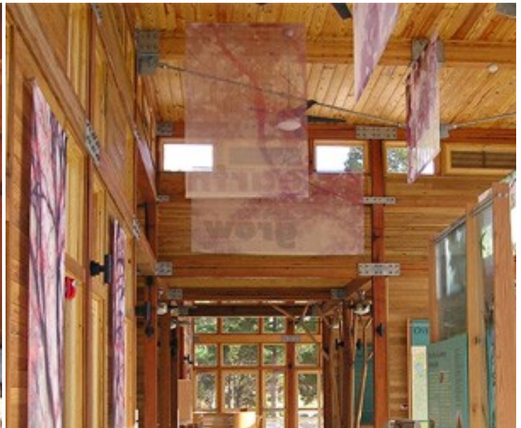
The Bernheim Arboretum Research and Visitors' Center used reclaimed materials, mechanical connections and reconfigurable modules to reduce waste and greenhouse gas emissions. Photo: Lifecycle Building Challenge via William McDonough + Partners
