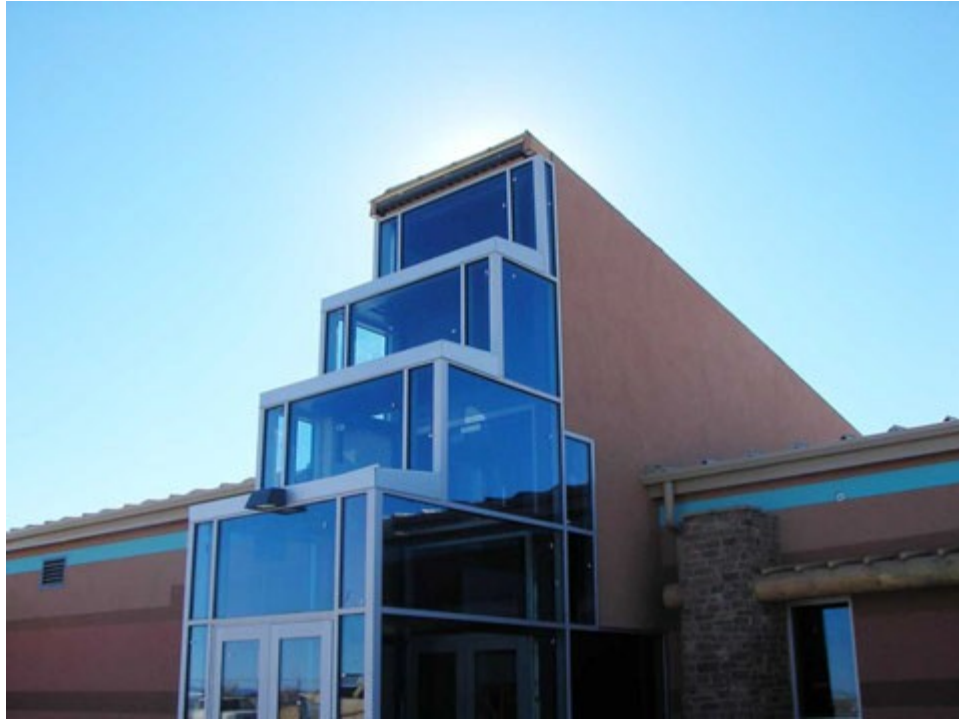
Kayenta Township, Navajo Nation, Arizona: Northeast Arizona Technical Institute for Vocational Education. Photo: Kayenta Township Building Department
